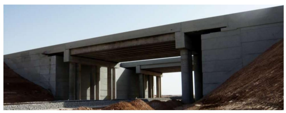
26 Overpasses: Bridges with Evergreen MAXI Bridge Abutments – This one for a Six Lane Highway
